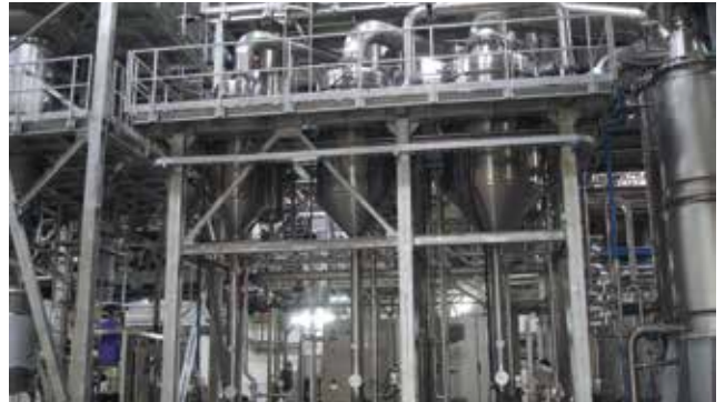
● COMPLETE INSTANT COFFEE PLANT INDONESIA, 2008
